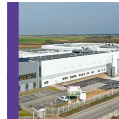
Blois (production site): LEED Gold ISO 14001 ISO 45001 ISO 50001
